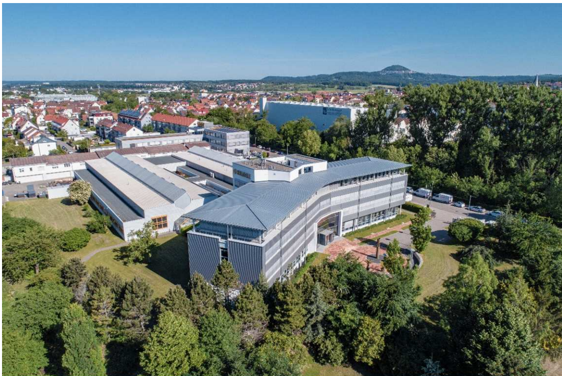
Firmengelände HELDELE GmbH © Tobias Fröhner Photography
