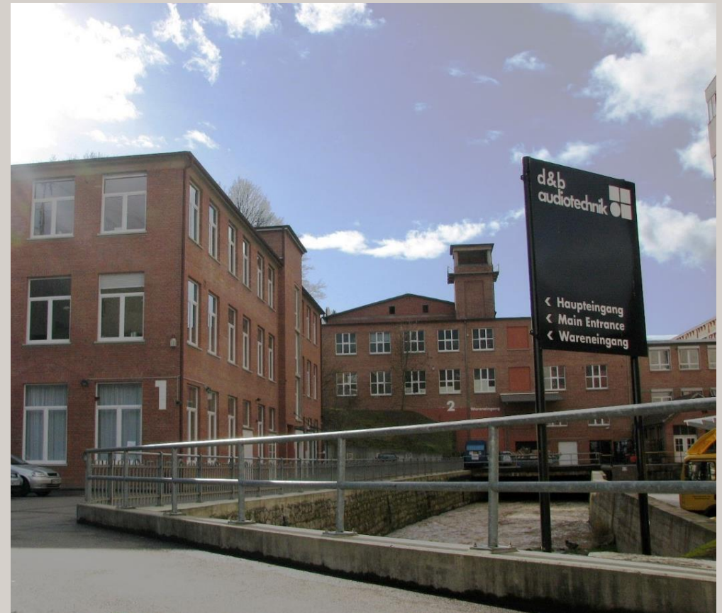
d&b Zentrale in Backnang
